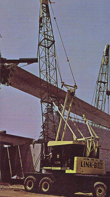
"Walking in" the "T" beams for the Gym was ticklish work.
