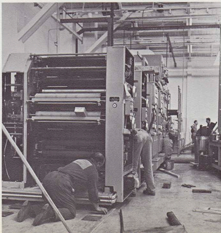
Lining up the four units of the web press was a tricky business.
